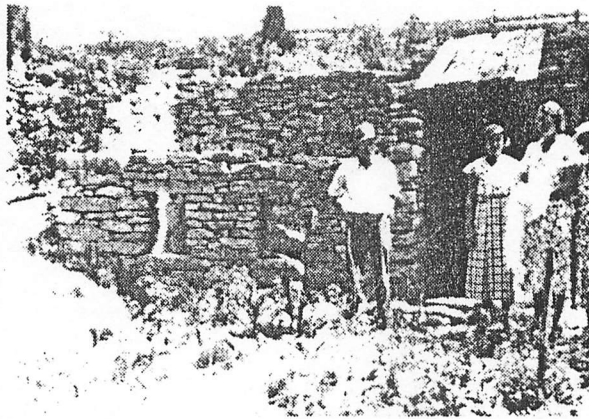
Today, The only visible remains of the Moravian Mission are the ruins of the Spring house built in the 1850's. This picture was taken in the 1940's. It has deteriorated considerably more since then.
